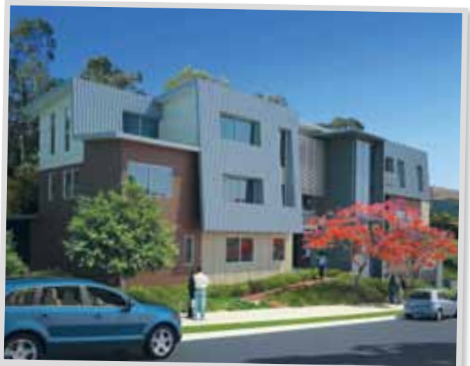
New ADAWS facility
