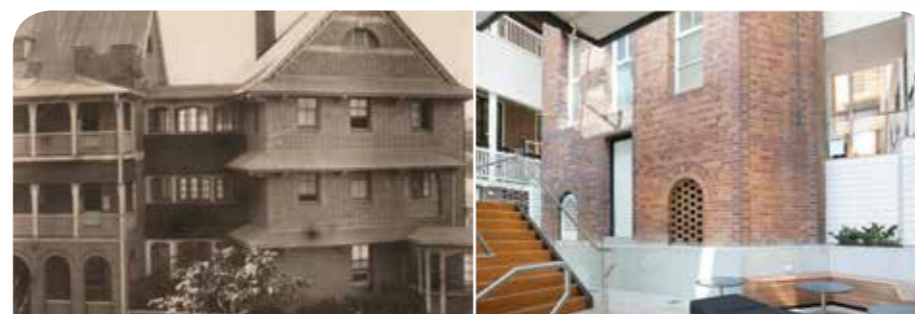
The Whitty Building when it opened in 1911, and in 2016 following its transformation into a unique education precinct.
