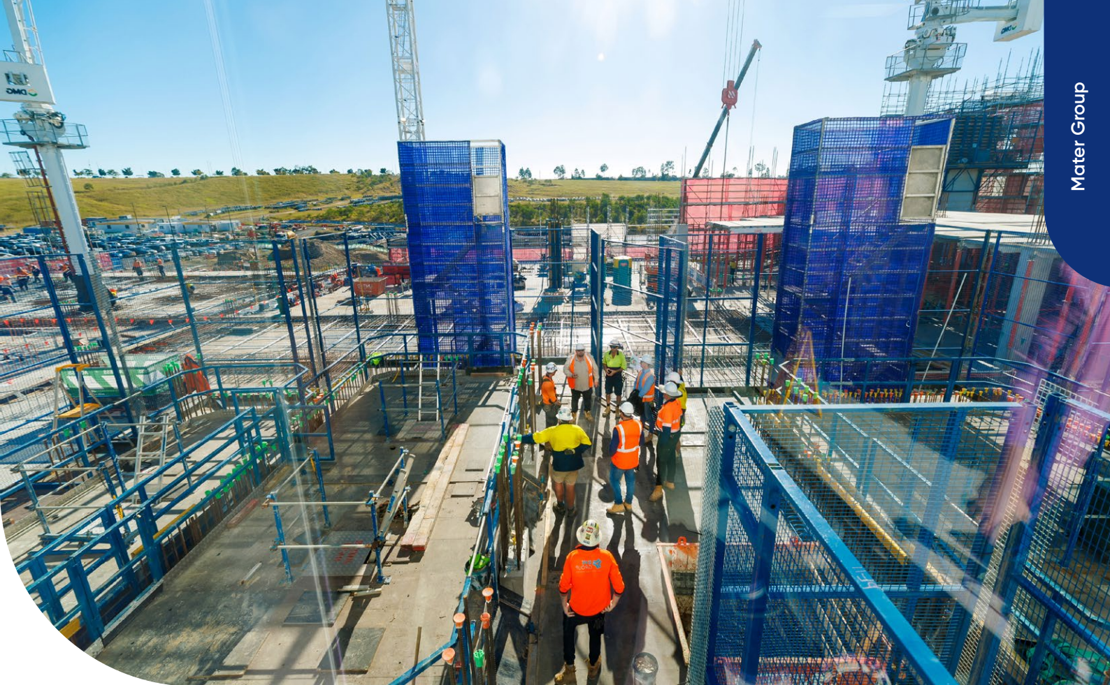
Mater Public Hospital Springfield construction
